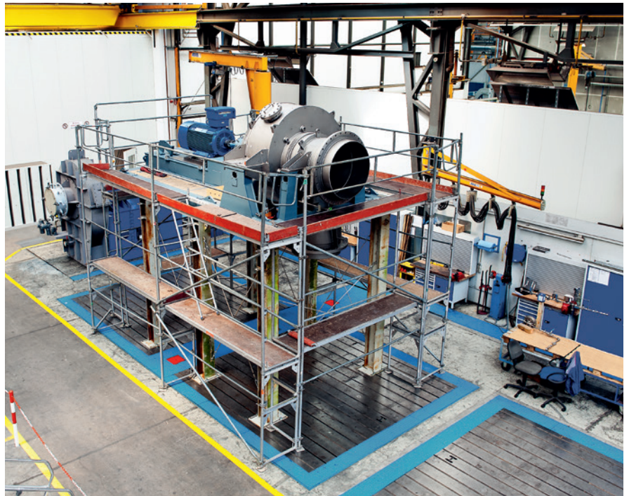
PILLER system testing field in Moringen, Germany
