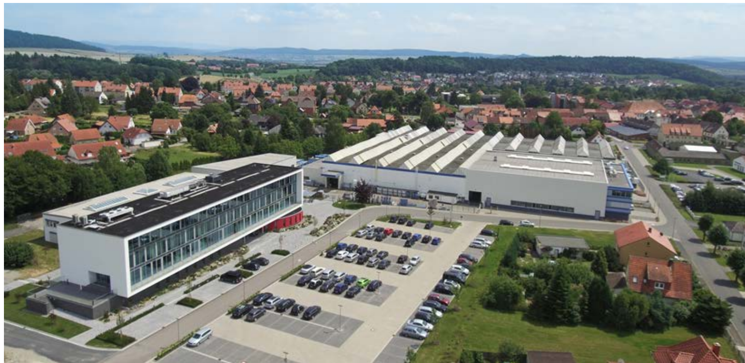
PILLER HEADQUARTERS IN GERMANY
